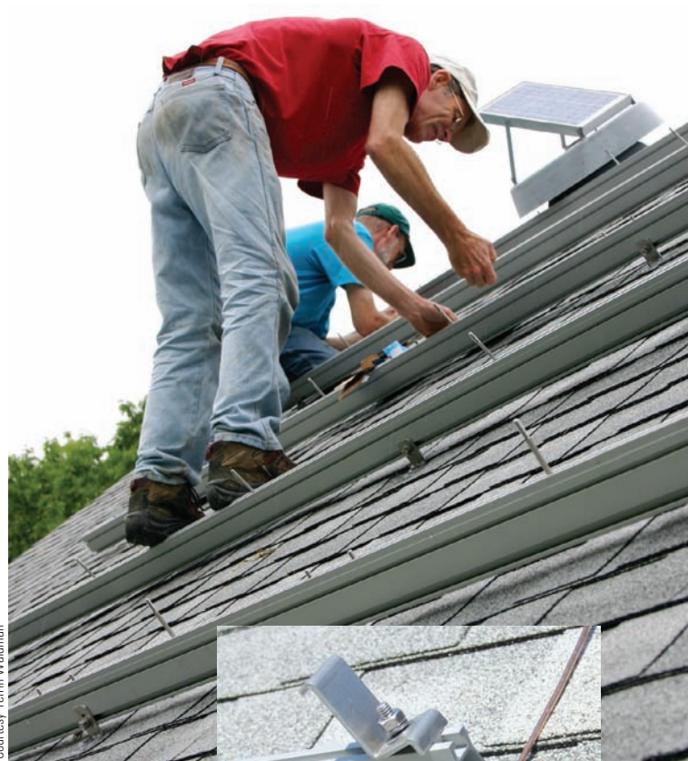
Above: The rails, installed and ready to receive the microinverters.
